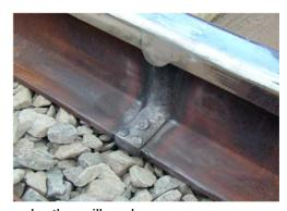
The SkV-T process was only introduced for 60E1/E2 rail profile, and in 2006 was superseded by the SkV-E process. The mould was withdrawn from use in 2007.
