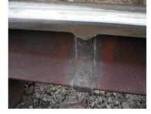
The SkV-E weld has a uniform weld collar approximately 40mm wide, and no re-enforcing rib under the head. (Note: If
