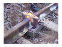
On completion of weld trimming, and not later than the time specified in Section 2, the excess head riser and mould is removed and placed in a safe position.
